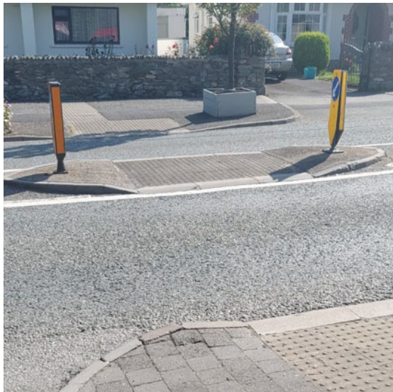
Figure 3 – Existing Uncontrolled Crossing
