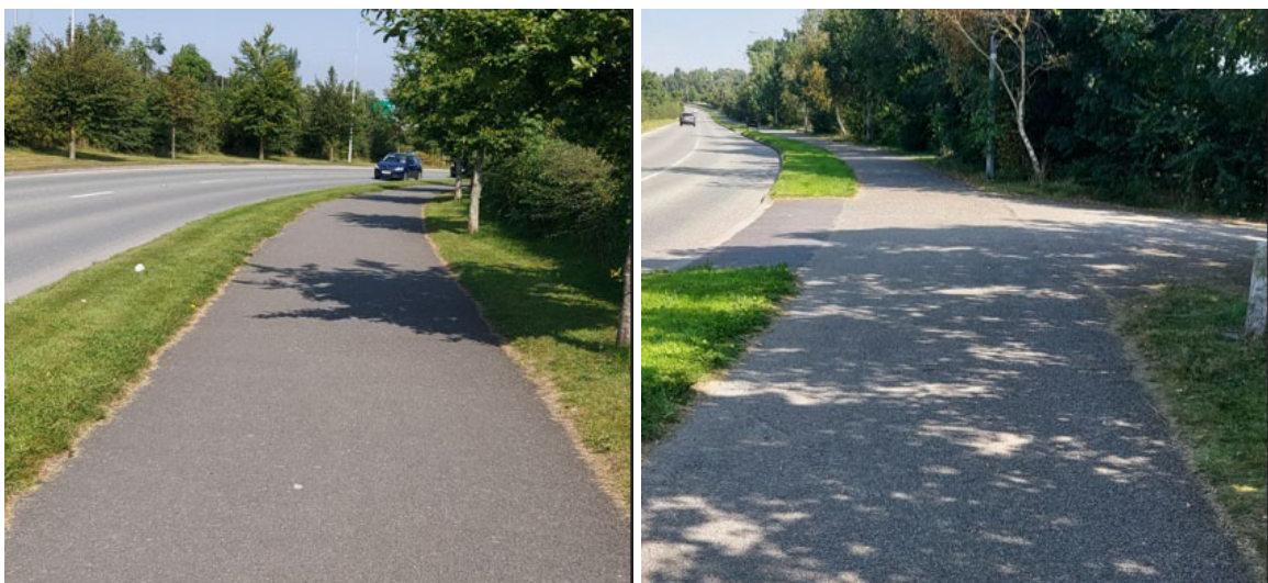
Figure 5 – Existing Shared Use Path
